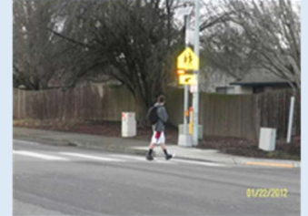
A RRFB is an active warning device used to alert motorists of crossing pedestrians. They remain dark until activated by pedestrians.
