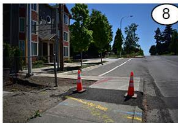
Two locations where relatively new development has built out an updated sidewalk. In both scenarios, the sidewalk has a tree-lined furnishing zone separating the walkway from motor vehicle traffic in the road. In #8, the sidewalk is set-back from the road and space is provided for parking or other curbside uses that operate outside of the travel lanes. (photos face south (#8) and north (#9))
