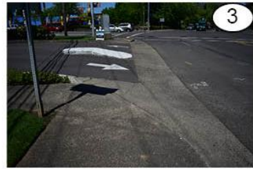
The driveway entrance just south of SW Hall Boulevard has a gap in the sidewalk and a splitter island defines direction of traffic for motorists. (photo faces north)
