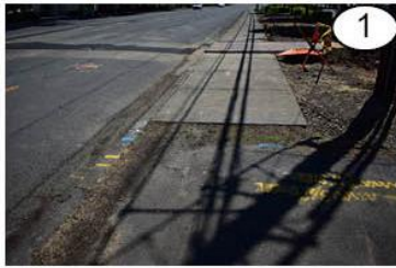
Conditions on the west side of the road, south of SW Hall Boulevard. (photo faces south)
