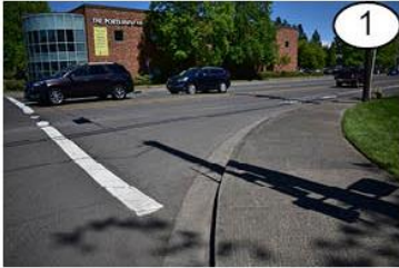
SW Hall Boulevard at the eastern leg of its intersection with SW Greenburg Road. The bike lane has been worn off and there is a large radius, accommodating high motor-ists speeds making the turn. (photo faces east)
