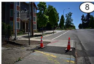
Two locations where relatively new development has built out an updated sidewalk. In both scenarios, the sidewalk has a tree-lined furnishing zone separating the walkway from motor vehicle traffic in the road. In #8, the sidewalk is set-back from the road and space is provided for parking or other curbside uses that operate outside of the travel lanes. (photos face south (#8) and north (#9))
