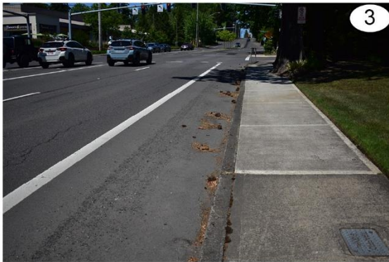
Debris in bike lane and multiple abandoned driveways (right) in sidewalk, compounding the debris issues. (photos face north)
