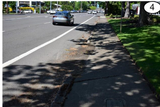
Debris in bike lane and multiple abandoned driveways (right) in sidewalk, compounding the debris issues. (photos face north)
