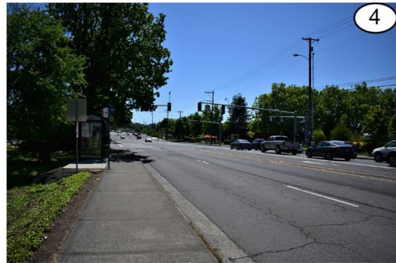
Bus stops on SW Greenburg Road at SW Washington Square Road (south). Northbound (left) stop has an additional paved waiting area behind the sidewalk. Both stops are accessible by sidewalk in both directions. (photo faces south)
