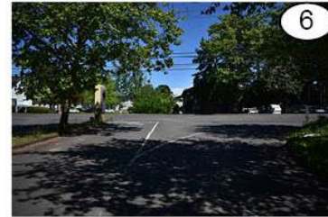
The approach to SW Greenburg Road from Summit Drive; the large curb radii accommodates high speed turning movements. (photo faces east)
