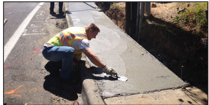
Tigard street crew fills a sidewalk gap.
