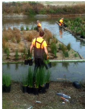
Launching and planting FTWs (photo courtesy Port of Vancouver)
