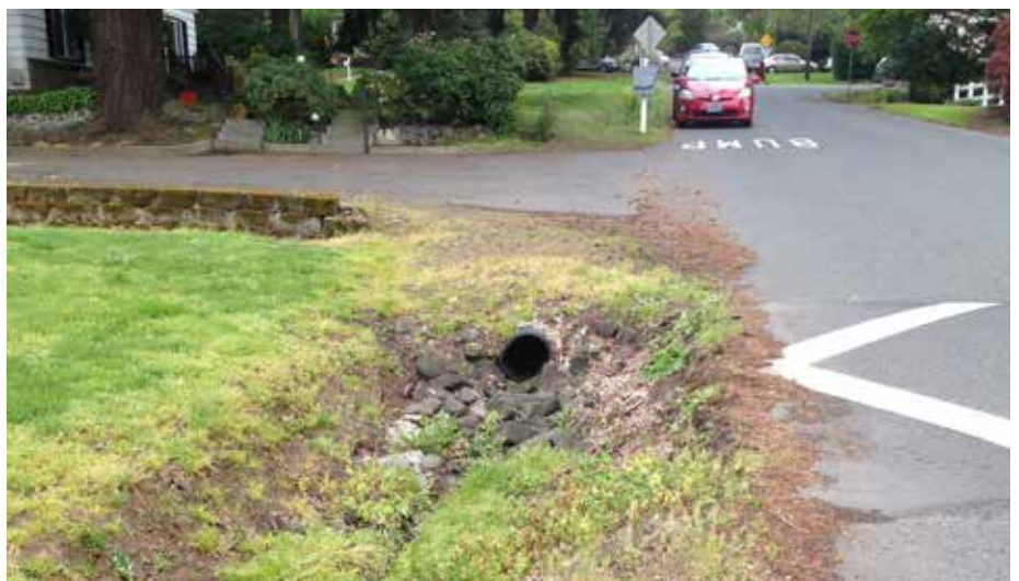
Open stormwater ditch along Baylor
