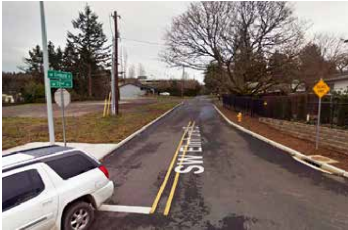
Left: Curbs and missing sidewalks along Elmhurst at 72nd | Right: Curbs and missing sidewalks along Hermoso
