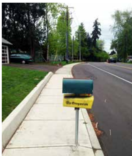
Mailbox along 72nd installed in new concrete sidewalk
