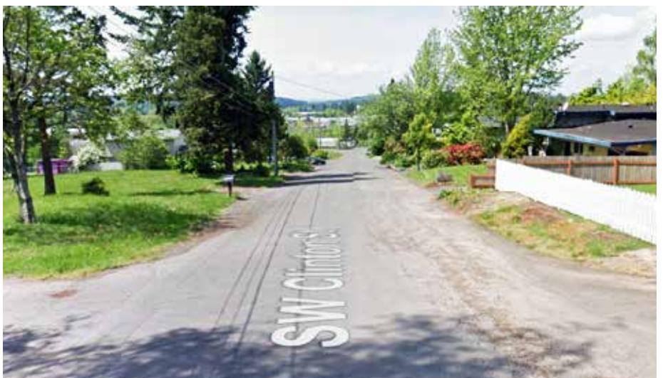
Missing sidewalks along Clinton near 70th
