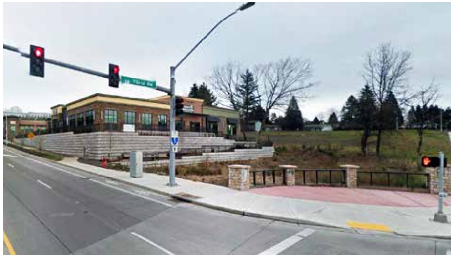
Special pavement treatment at a plaza at the intersection at Dartmouth and 72nd
