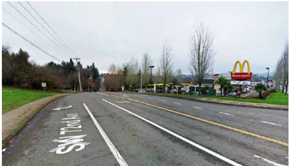
Steeper grades along 72nd Avenue north of the Red Rock Creek
