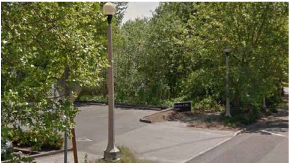
Pedestrian-scale lighting along 74th near 99W/Pacific Highway
