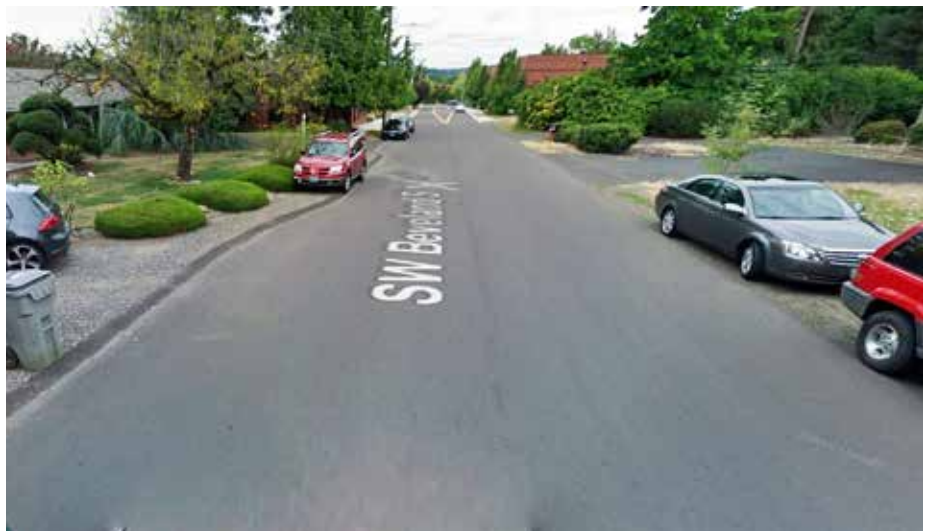
Missing sidewalks on both sides along Beveland near 70th
