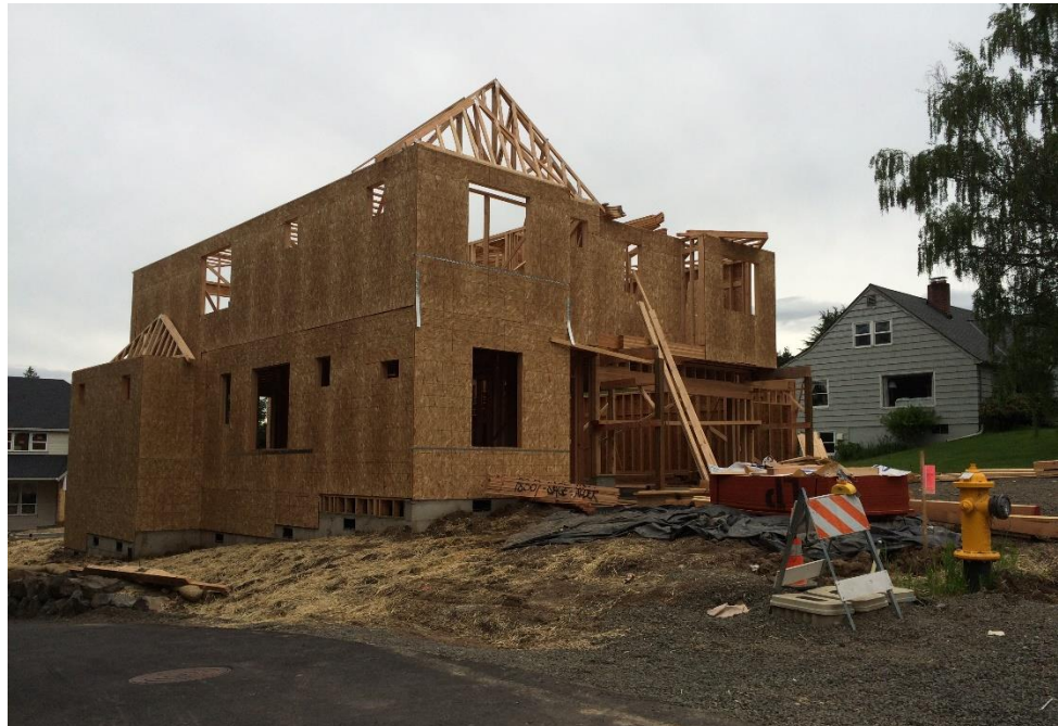
New housing construction in Tigard
